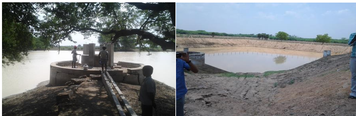
Image 3. Renovated Ranisethupuram Oorani with a bore well in Ramanathapuram District, Tamil Nadu
