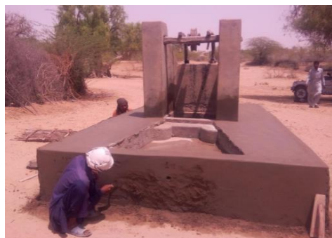
Image 3. Well restoration in progress
